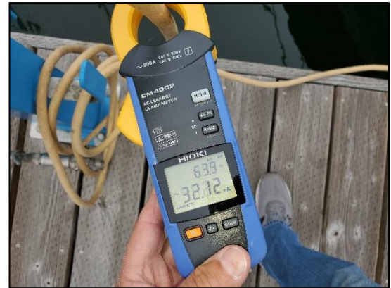
NFPA 303 requires a fault current test prior to plugging into a non-ELCI protected marina
