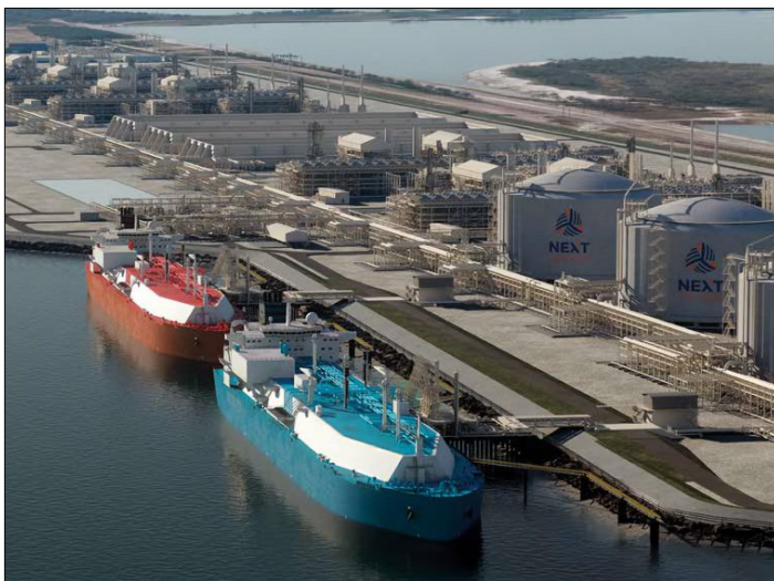
Figure 10: An illustration of the Rio Grande LNG's 984-acre facility courtesy Port of Brownsville/NextDecade
